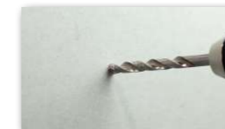
1 Ø 10 mm Loch bohren.
